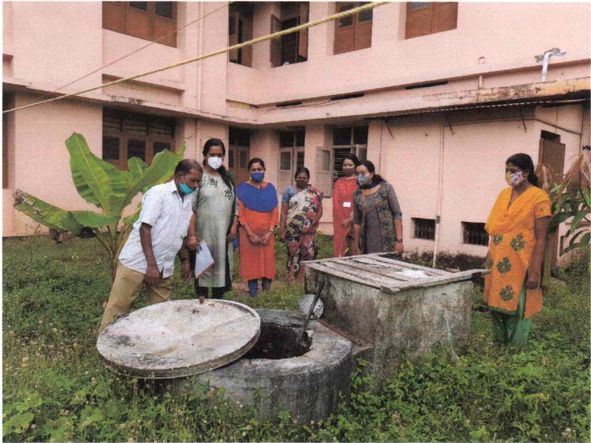
BIOGAS PLANT IN THE HOSTEL
